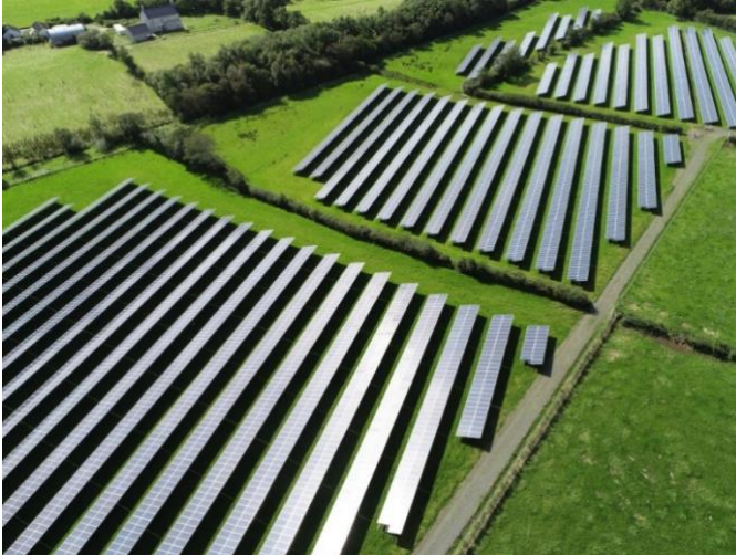
Lough Road Solar Farm; Greencoat Solar Fund II
